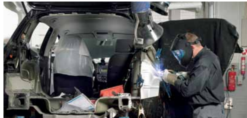
MIG/MAG welding in sheet metal
